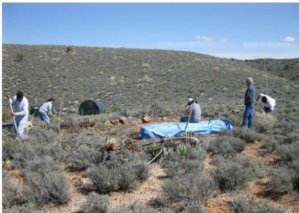
Figure 1. An apron catchment construction catches rain and snow to collect water for wildlife and cattle on the Hualapai Indian Reservation
